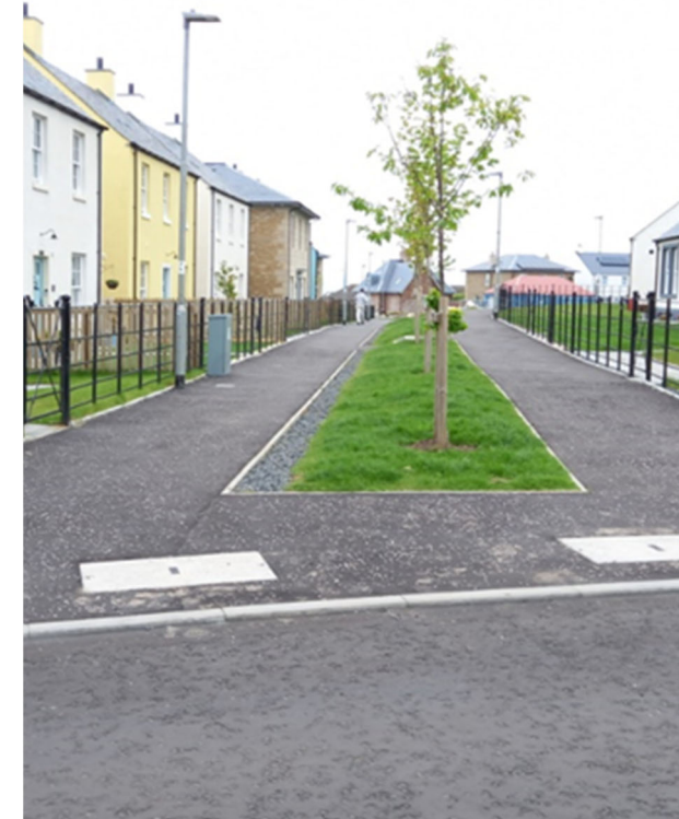
Figure 2 – Filter Trench for Rainwater Management
